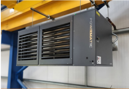
New Warm Air Heaters supplied & installed
